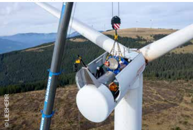
Mobile crane erects a wind turbine in eastern Austria.
